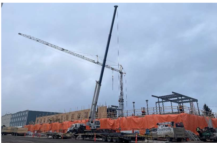
Pre-fabricated framing panels being installed on Hyatt Place site.
